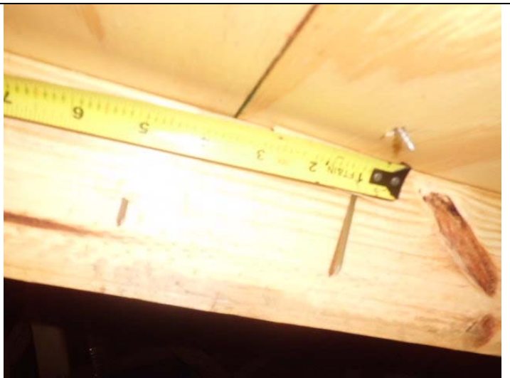
Roof deck attachment
