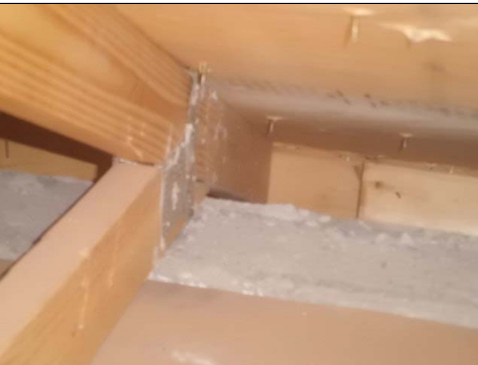
Roof to wall attachment
