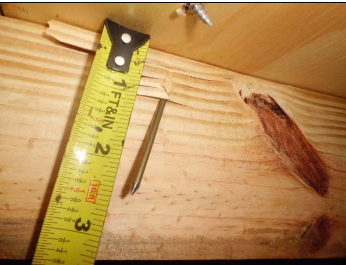
Roof deck attachment
