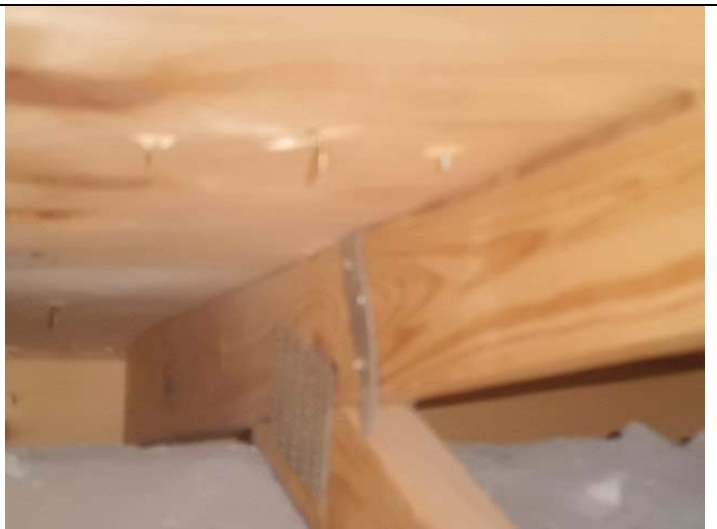
Roof to wall attachment
